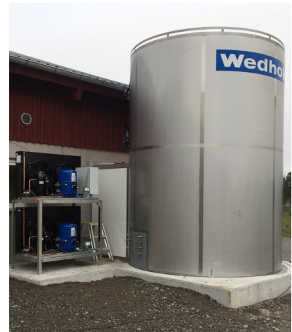
Silo with cooling unit and alcove during installation.
